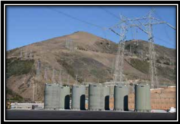
Dry Cask Storage
